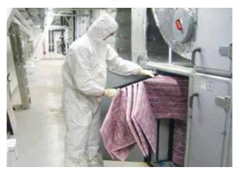
Figure 9: Personal protection equipment for filter replacement
